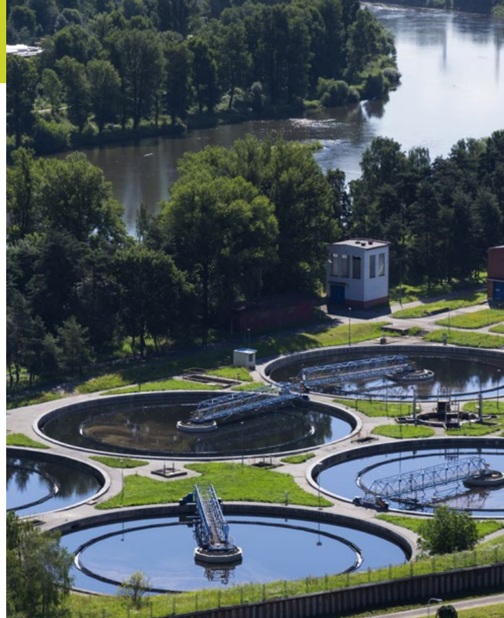
Aerial view of storage tanks in sewage water treatment plant
