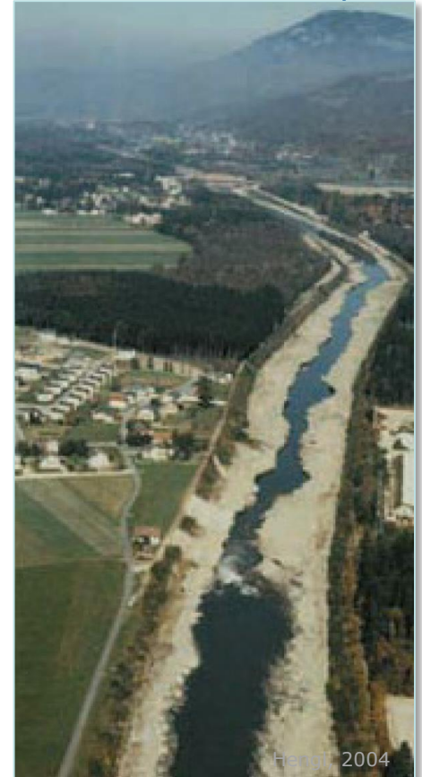
Interruption of sediment transport
