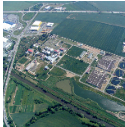
Wastewater treatment plant Brno-Modřice
