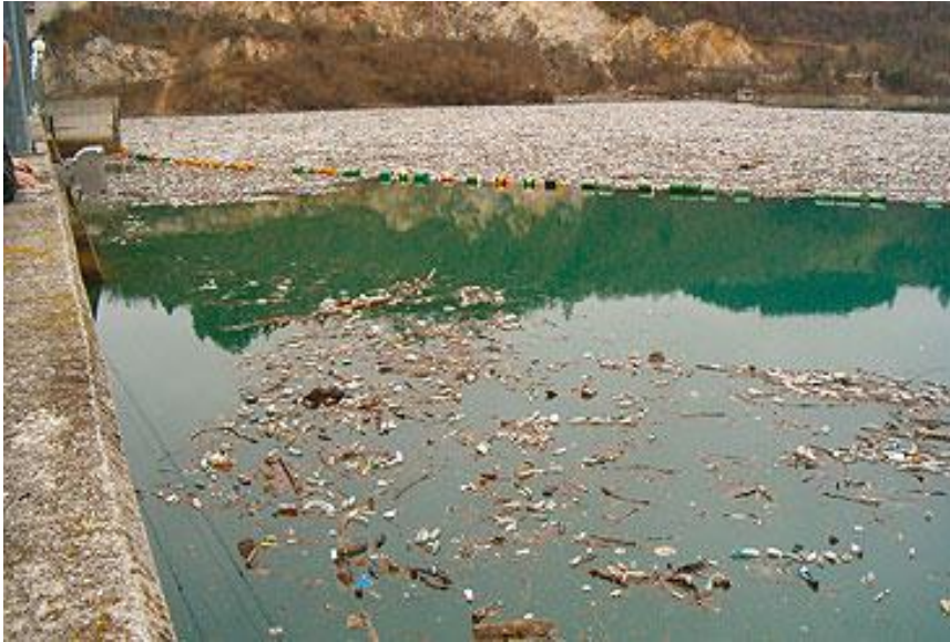
Flooding waste backs up behind the dam of the Višegrad power plant on the Drina River (a tributary of the Sava River within the Danube River Basin).
