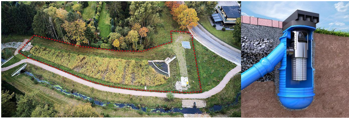
Figure 13 Retention soil filter on Manshardtstraße (42)
