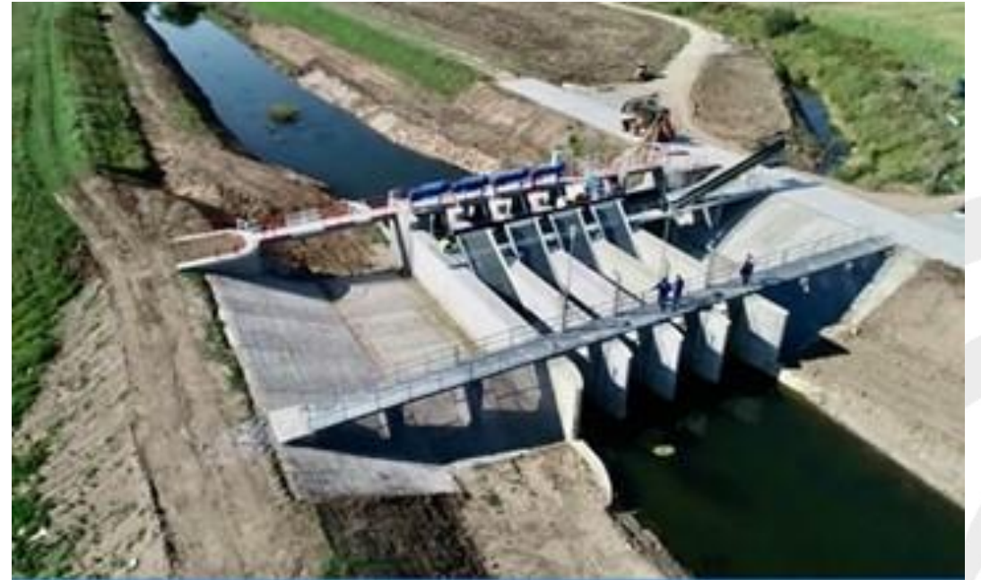
12 waste barriers on tributaries of Tisza
