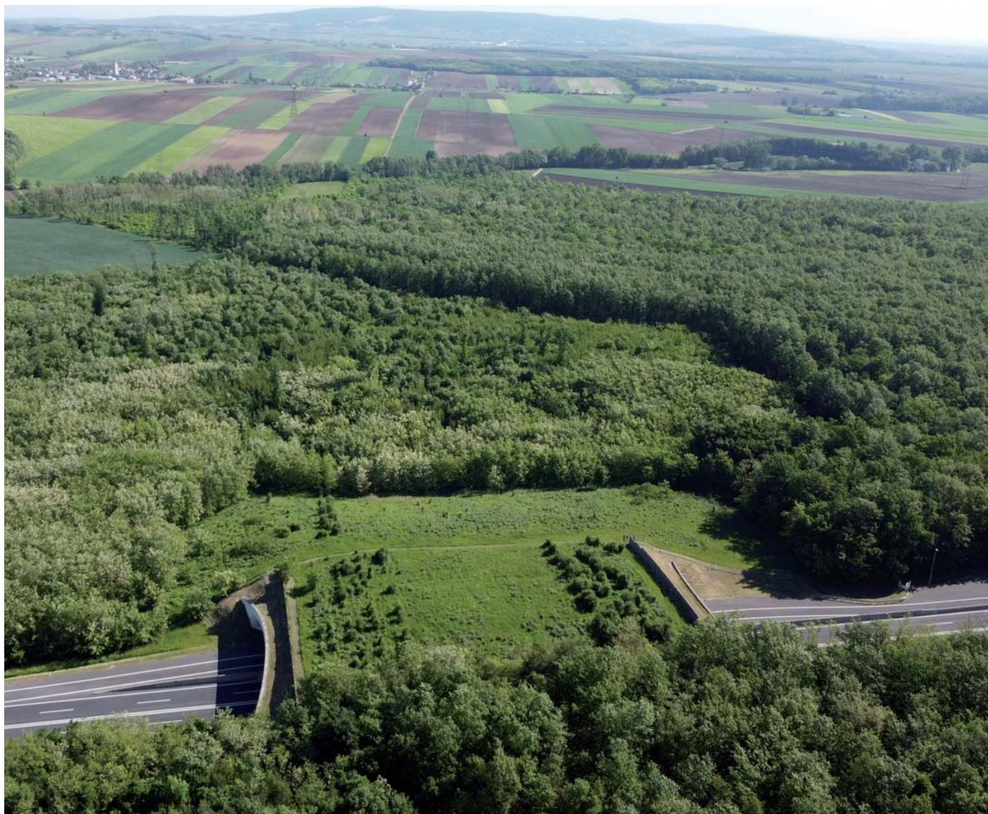
Green bridge near Pöttsching, Alpine-Carpathian corridor, copyright: Gebhard Banko, Environment Agency Austria.
