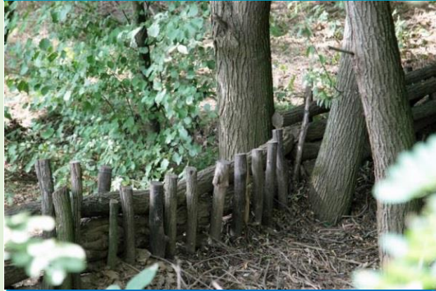
Slowing the flow with leaky wooden dams
